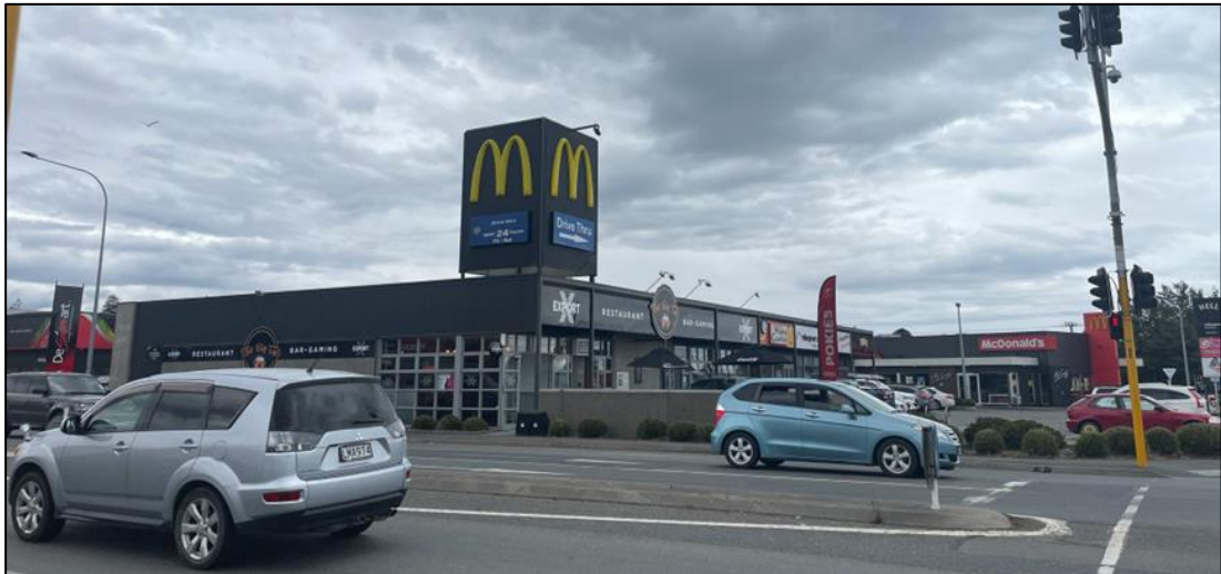
Figure 4 Businesses and associated signage operating in the north-western corner of the adjacent intersection, with signage installed above the parapet (TPG)
