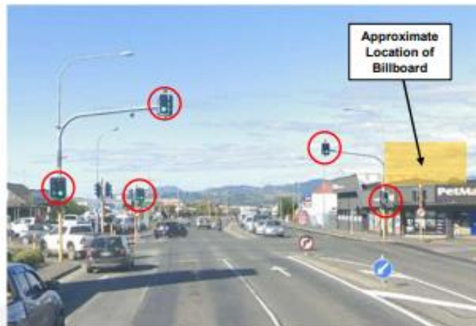
Photograph 6: Traffic Signal Locations on Gladstone Road in Relation to Billboard Location
