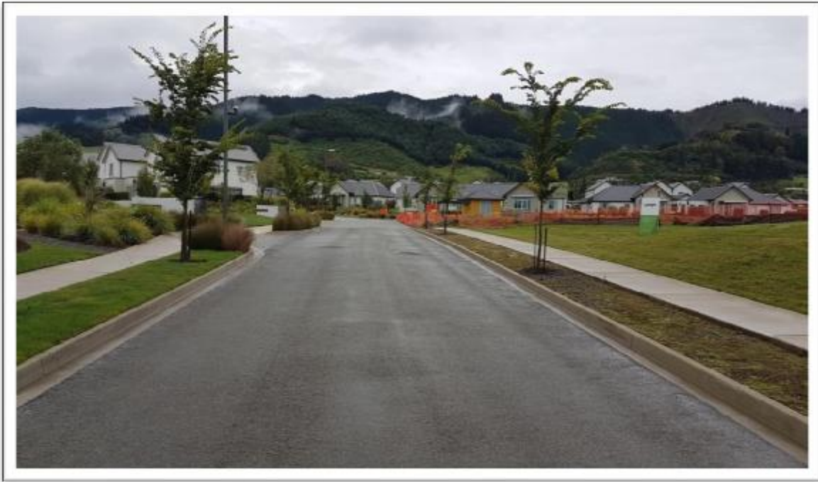
Figure 6: A specifically designed Collector Road
