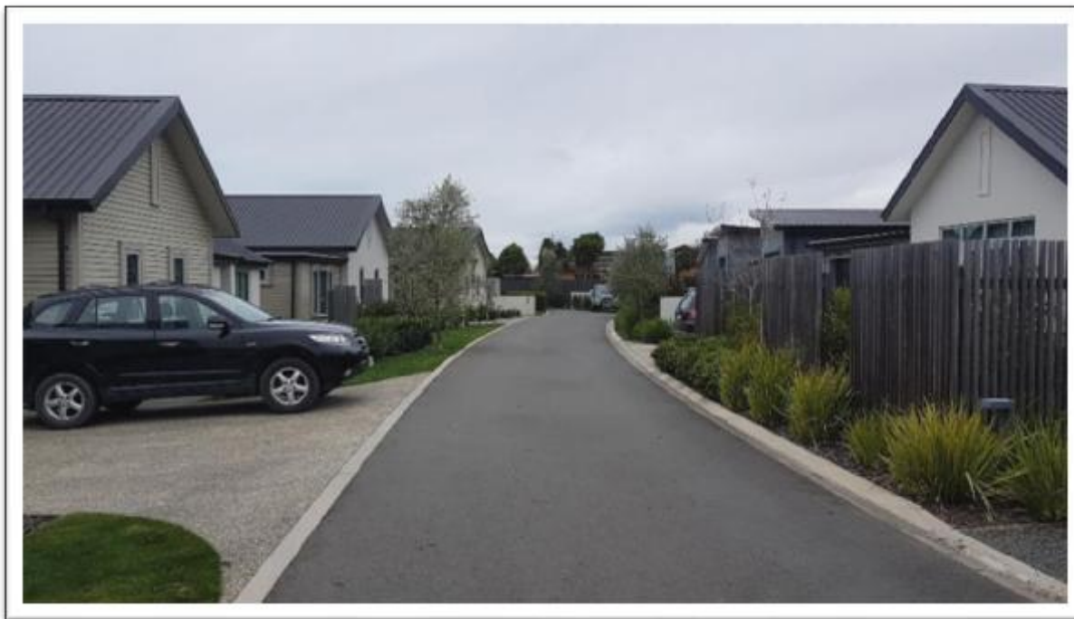
Figure 9: Access Place (4.0 metres)
