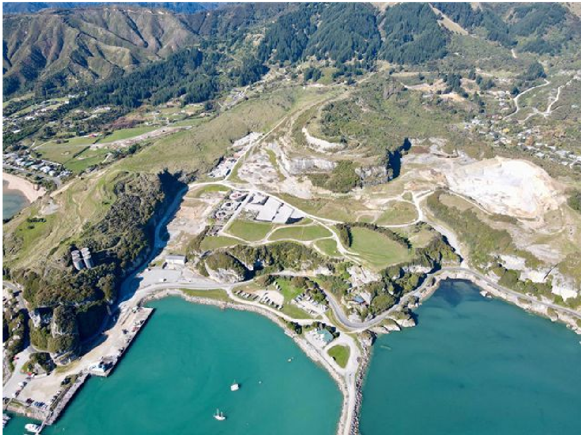
Photo 1: Aerial view of the Port and surrounding land at Tarohe, Eastern Golden Bay.
